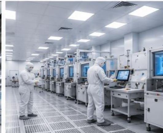
MISSION-CRITICAL ENVIRONMENTS (CLEANROOM)
